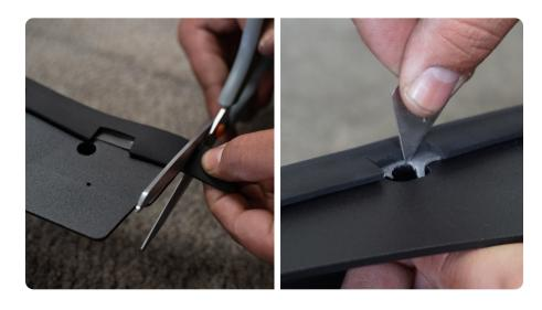
STEP 11 | Hold up the fenders to the vehicle and note what holes will be used. Install the provided nutserts using a nutsert tool. If you do not own a nutsert tool, we provide one with our kit.
